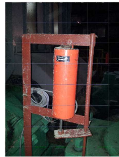
Mill Top Roller Lift Sensed Installation
